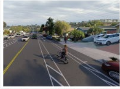
Widened sidewalks and buffered bike lanes on Kelly Drive from El Camino Real to Hillside Drive
