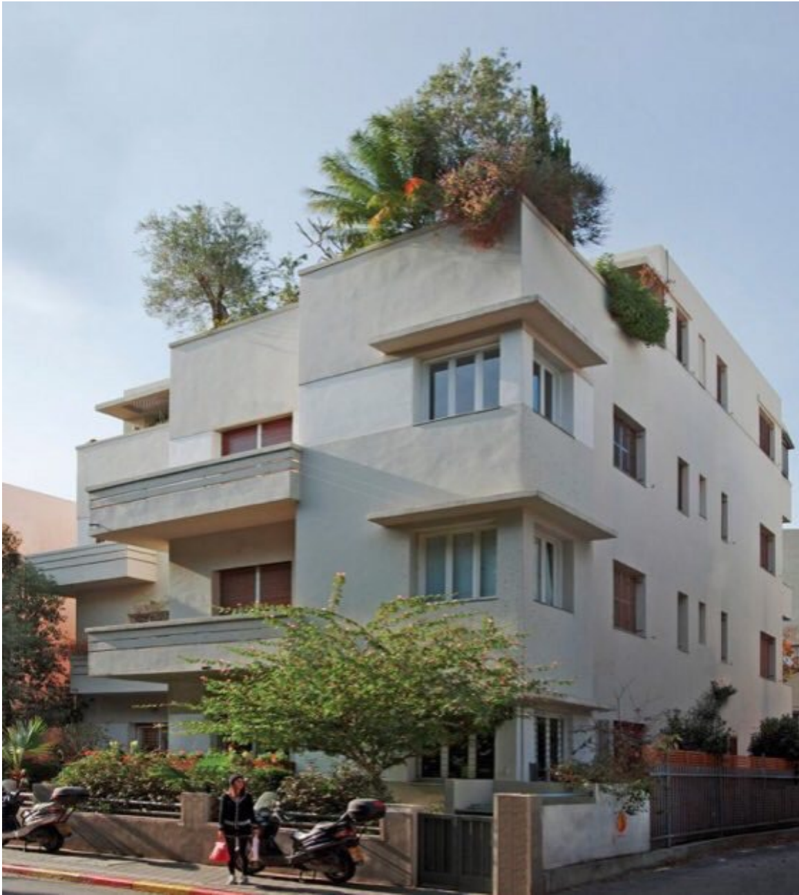
Roof Patterns and Architecture Style
