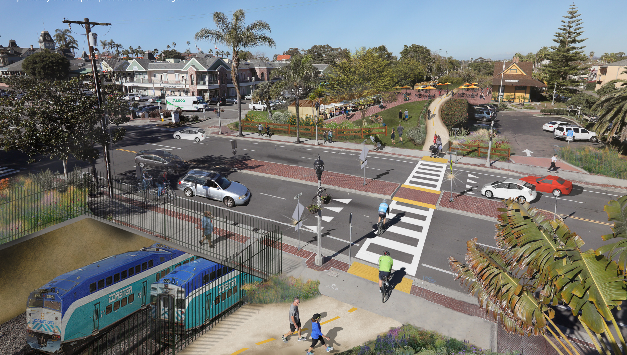
Future double tracks in a trench, below street level with a possibility to add open space at Carlsbad Village Drive
