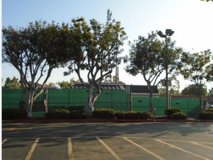
Exhibit 5. Building 4, primary (southwest) elevation, view to east.
