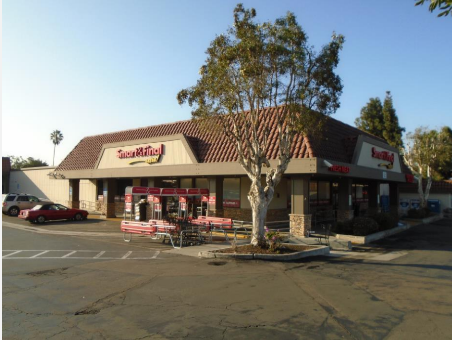
Exhibit 2. Building 1, primary (northwest) and northeast elevations, view to the south.
