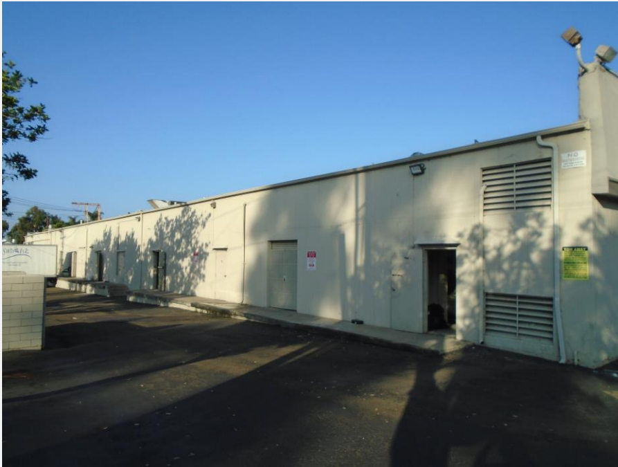
Exhibit 3. Building 1, rear (southeast) elevation, view to the west.
