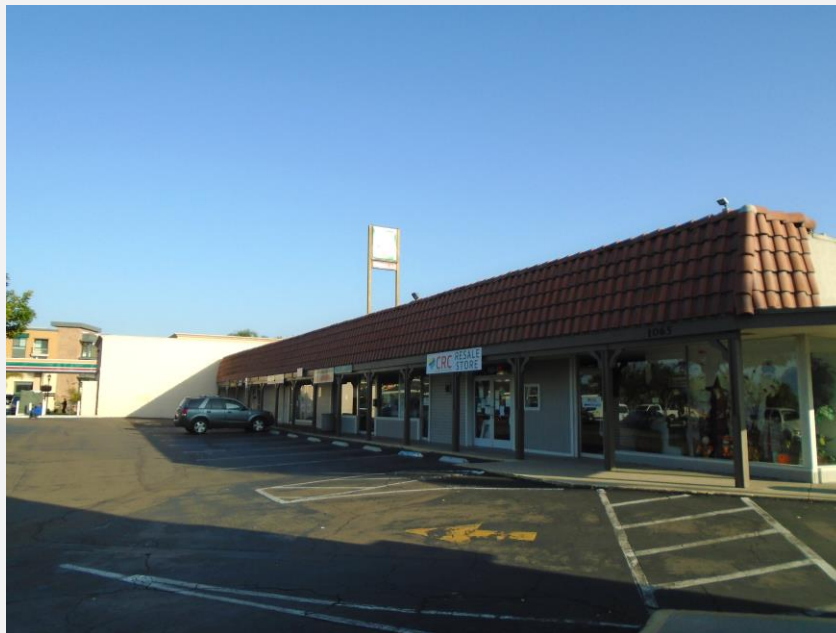
Exhibit 5. Building 3, primary (southwest) elevation, view to the north.
