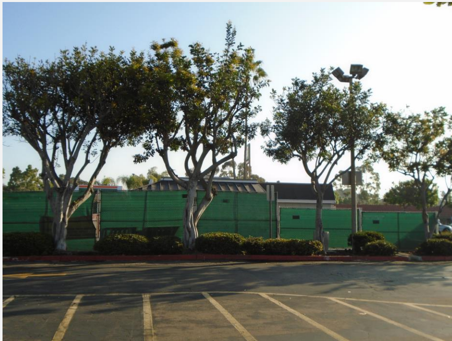
Exhibit 6. Building 4, primary (southwest) elevation, view to east.
