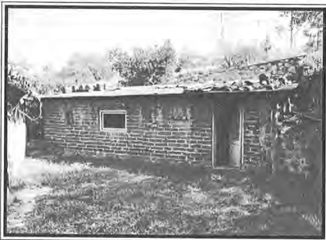
Garage at caretakers house
