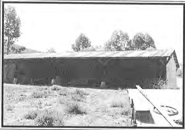
Equipment shed and blacksmith's shop
