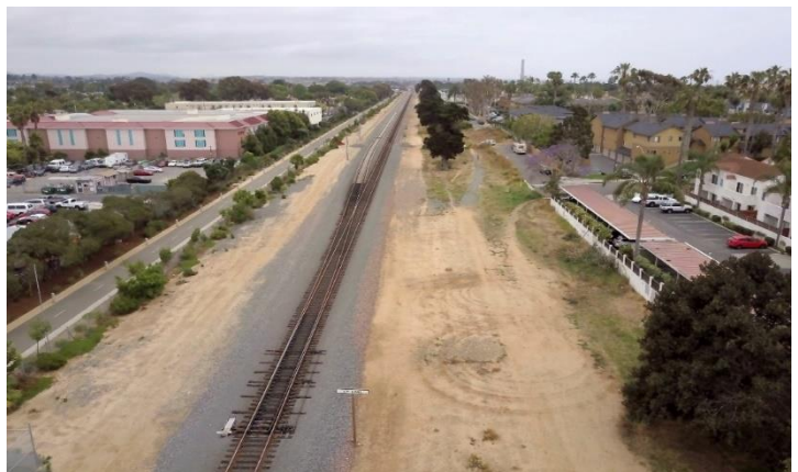
NCTD Rail Corridor – Potential to add more parking as a shared resource
