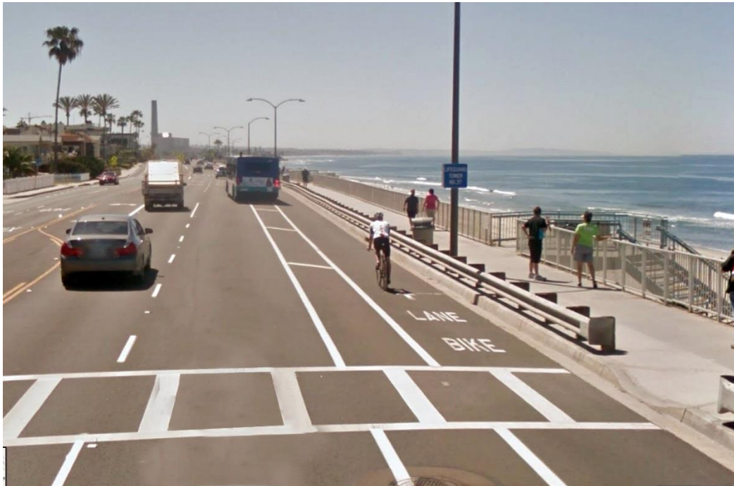
Buffered bike lane along Carlsbad Boulevard
